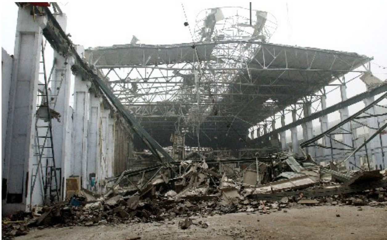
1 Figure 2 – Ground level view of a casthouse following a molten metal explosion
