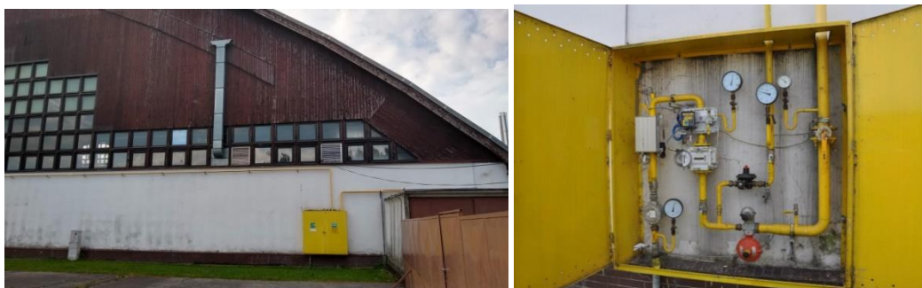
Obr. 6: Meranie spotreby plynu
