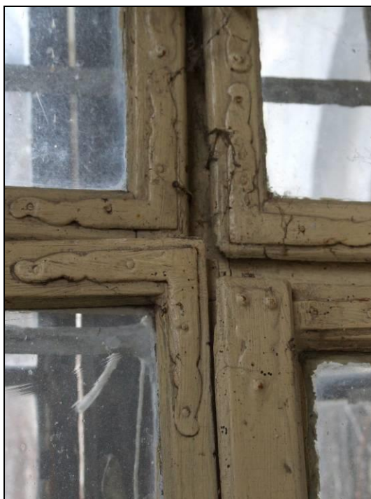
Detail uholníkov a klapacej lišty.
