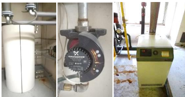
Obr. 11: Ohrev TV, kotol K9
