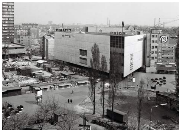
OD Prior počas výstavby (foto: 4dny http://bit.ly/1TC145H ) The Prior department store during construction (photo: Four Days http://bit.ly/1TC145H )
