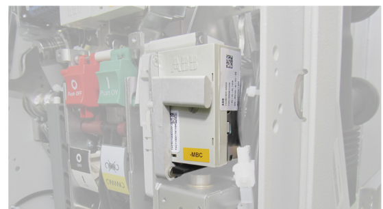
MBC : Shunt closing release
