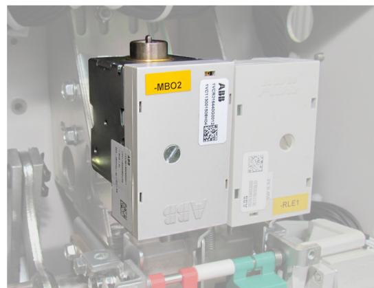
MBO2: Additional shunt opening release
