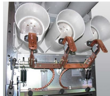
Insulating monoblocks with contacts for rated current up to 2500 A.
