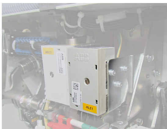
RLE1: Locking magnet on operating mechanism
