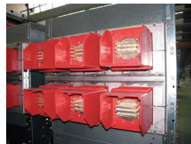
Insulating monoblocks with contacts for rated current of up to 4000 A.
